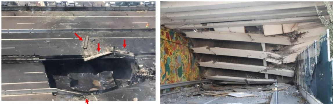
Figure 7: Structural effects in the epicenter of the explosion
