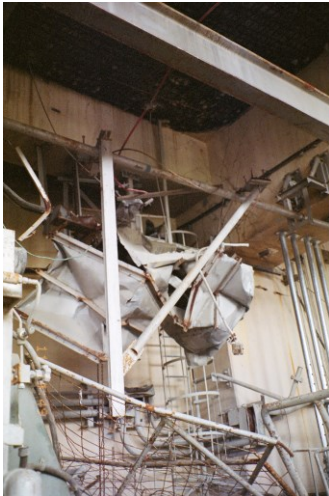
Figure 1 Damaged Duct
