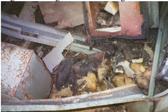
Figure 3 Black colored insulators near an MG set
