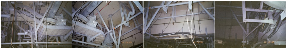
Figure 11 Fragments on cable rack
