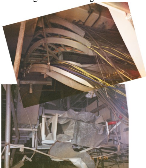
Figure 7 Duct (lower) and cable rack (upper) damage
